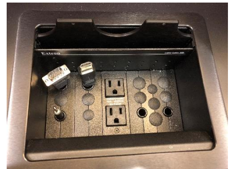
Cable Cubby showing VGA/HDMI/audio cables
